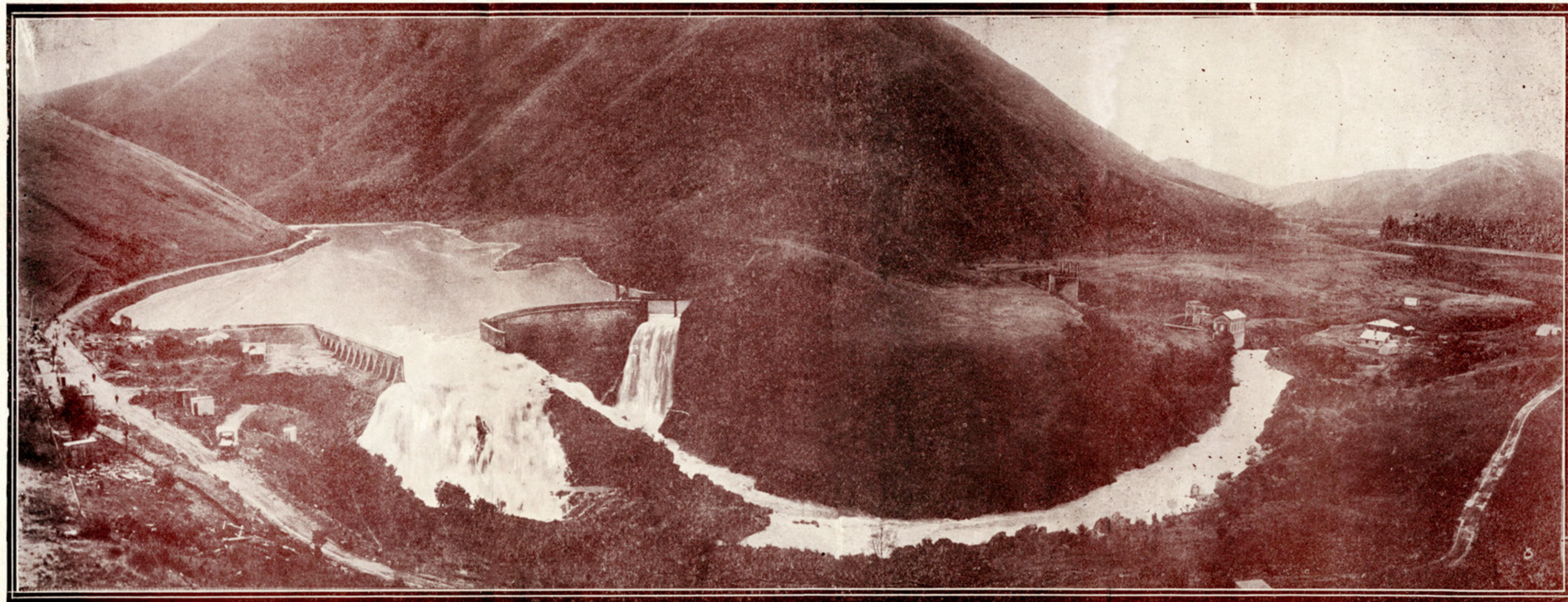
A COMPREHENSIVE PHOTOGRAPH, SHOWING THE WHOLE OF THE WORK CARRIED OUT BY THE MARLBOROUGH ELECTRIC POWER BOARD IN HARNESSING THE WAIHOPAI RIVER.
