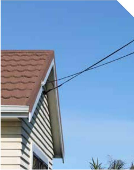
A reminder that property owners are responsible for the power line from the point of supply, which is normally where the line crosses the boundary of the property to the point of connection to the installation. This is typically known as the service line. However in some areas, especially rural areas, the point of entry to a property might not be clear. If you are not sure which portion of the power line is your responsibility, please contact Marlborough Lines.
