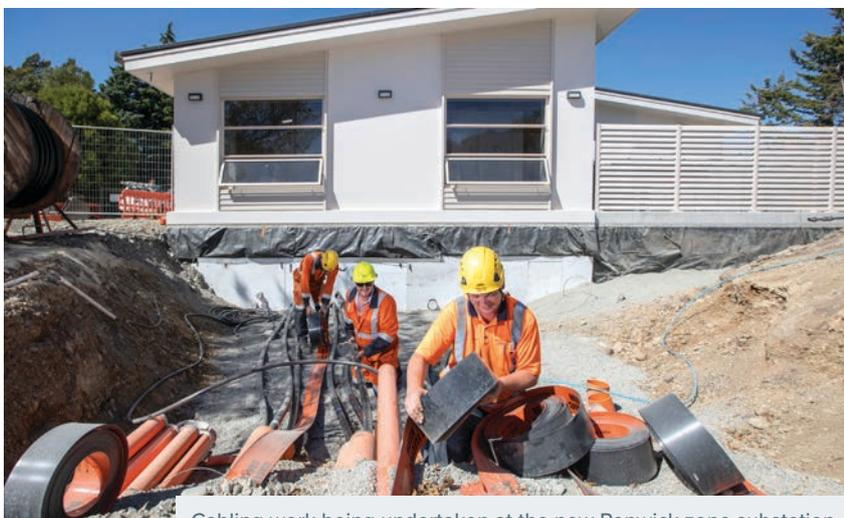
Cabling work being undertaken at the new Renwick zone substation
